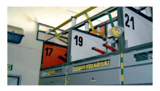
Short circuit duration: 0,04 seconds Short circuit current: 8kA Effects: No arcing damage. Need to replace a broken support insulator.
